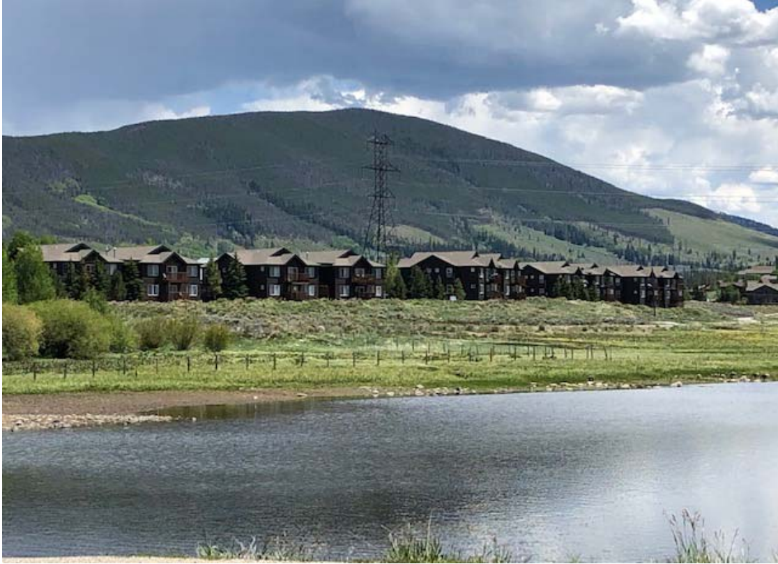
View of Project From Swan Mountain Road
